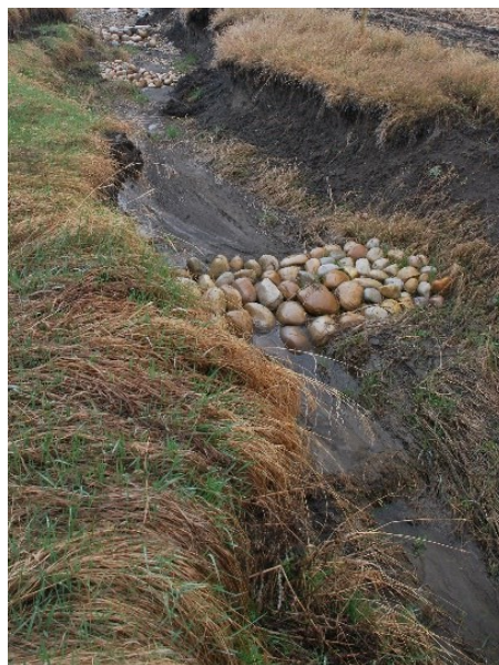
Left: One rock dam being constructed by volunteers in the September 2018 workshop.
